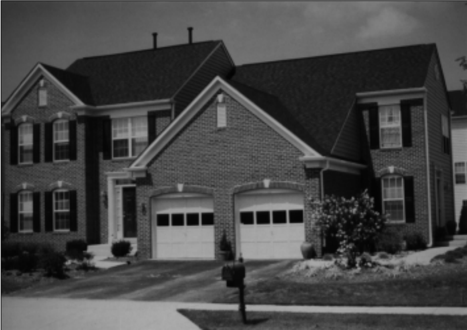
This house holds two Moderately Priced Dwelling Units. Note the front entrance (left) and side entrance (right).
